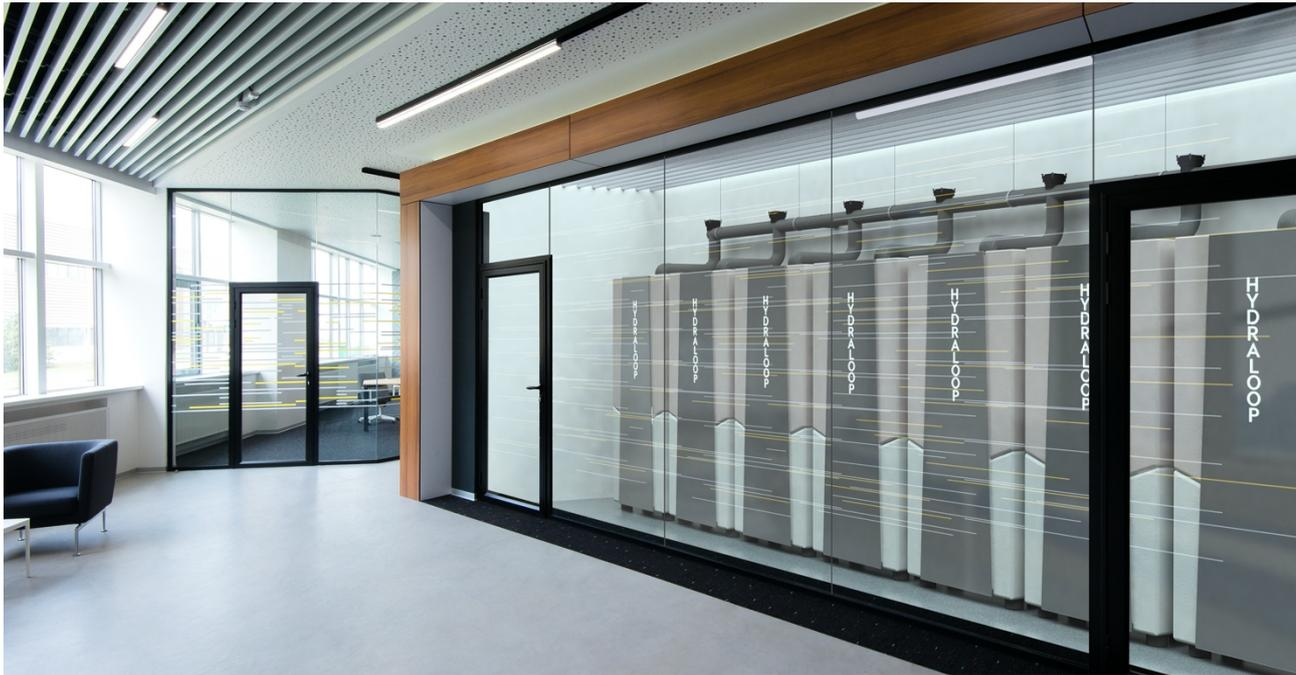
With the scalable and made to measure Hydralooop Cascade system, you can recycle up to 95% of shower, bath and/or handbasin water + the cooling water from air-conditioning units. Due to its innovative and breakthrough technology the maintenance requirements and corresponding costs are very low.
